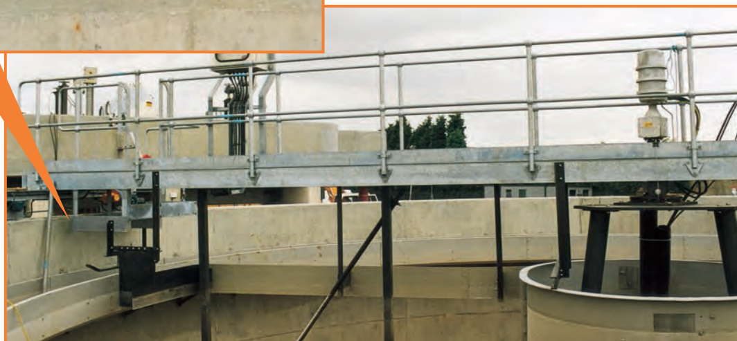
Half Bridge scraper for rotary settlement tank
