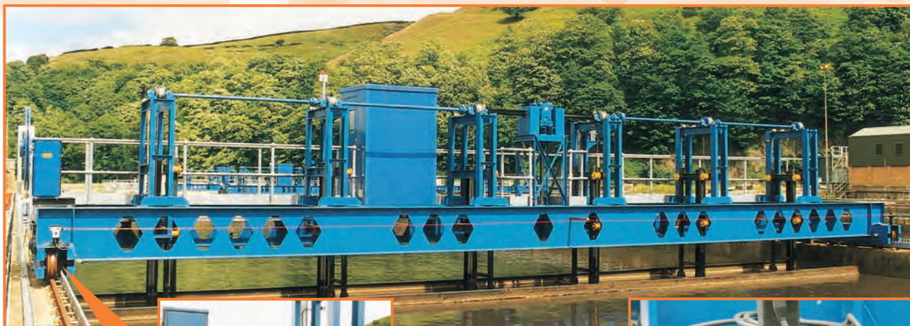
Bridge scraper for rectangular settlement tank
